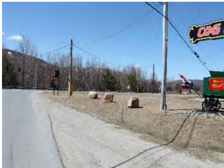
Photo 2-2 indicates an area in which excavation was performed but no markings by AWC are shown. Puc 800 rules require markings of any underground water mains within established tolerance zones or provide positive response that no water mains are present within the tolerance zone.
