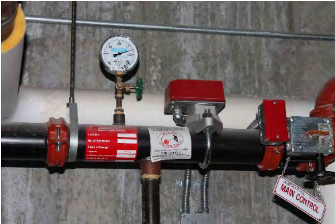
Photo #5-04 View of a Mt. Washington hotel fire sprinkler system pressure gauge noting 225 psi.
