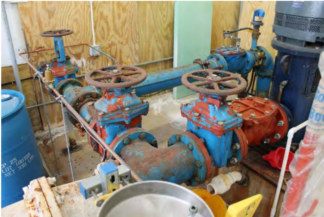
Photo #5-01 Depicts corrosion of pump station piping components.
