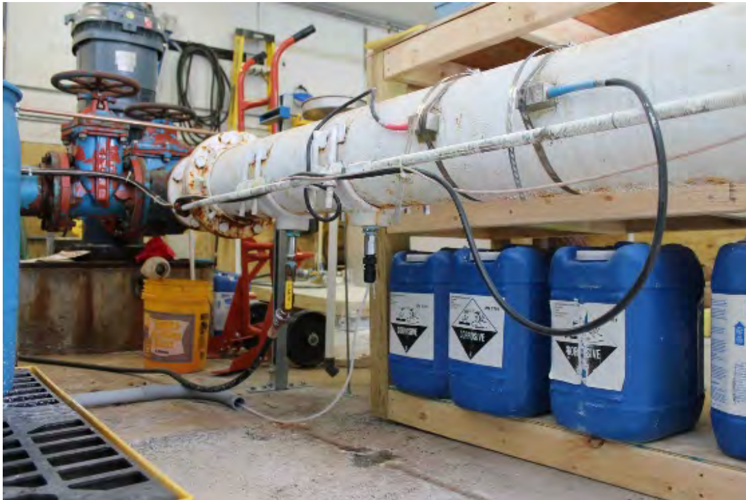
Photo #5-06 View of pump station components with stored corrosive chemicals, creating corrosive atmospheric environment.
